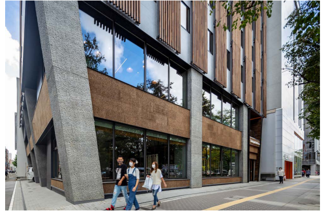
The lower levels on the north and east sides have large windows facing Odori Park.
