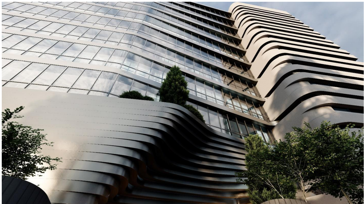
Image 4. the use of horizontal and jagged lines in facade design
