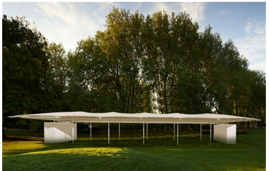
MPAVILION 2019, DESIGNED BY GLENN MURCUTT AO University Square, University of Melbourne
