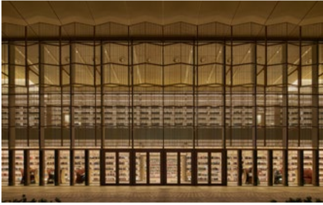
Perforated aluminium sun screens © Chris Goldstraw
