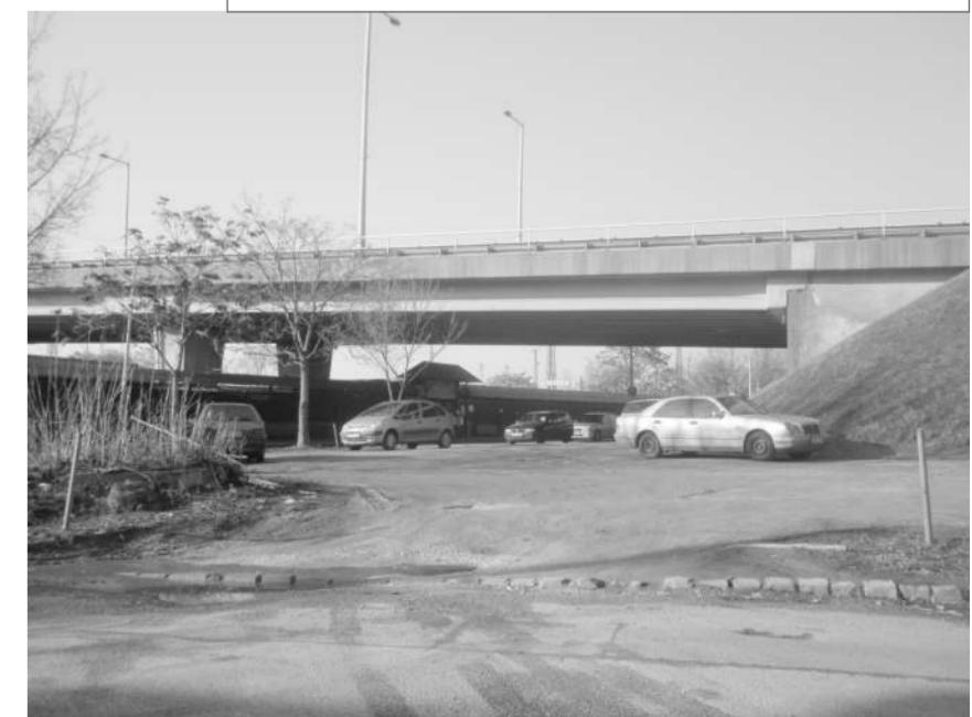
view of the market under the bridge
