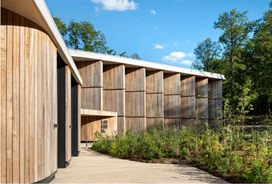
Like the basement, the roof too is in concrete, but vegetalised. Floor to ceiling glass on each level assures the interiors panoramic connection to the hotels immediate environment and regional views beyond. Clad in wood, the building is an architectural and cultural extension of the surrounding forest.
