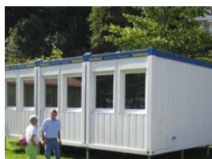
Office container buildings
