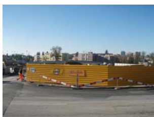
Construction site fences
