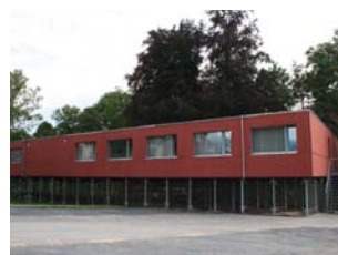
Container systems on piers
