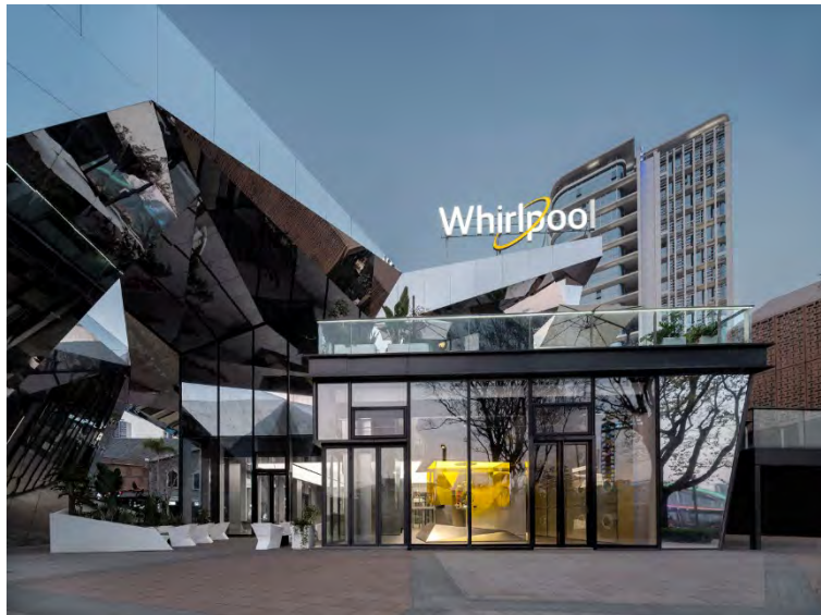
View from exterior to interior
