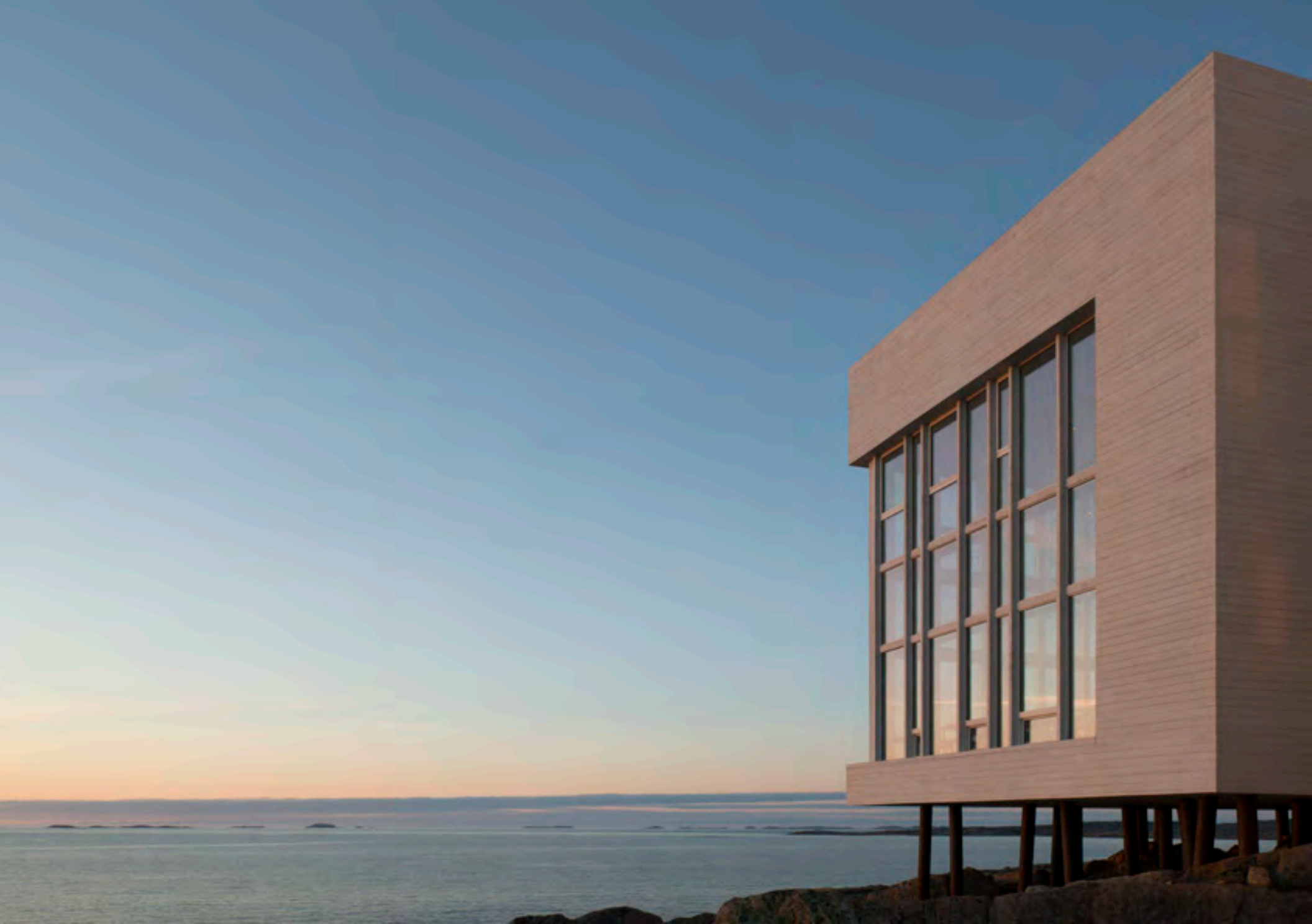
The dining room with Little Fogo Islands in the distance / FII_Architecture_5516_photo_Alex_Fradkin
