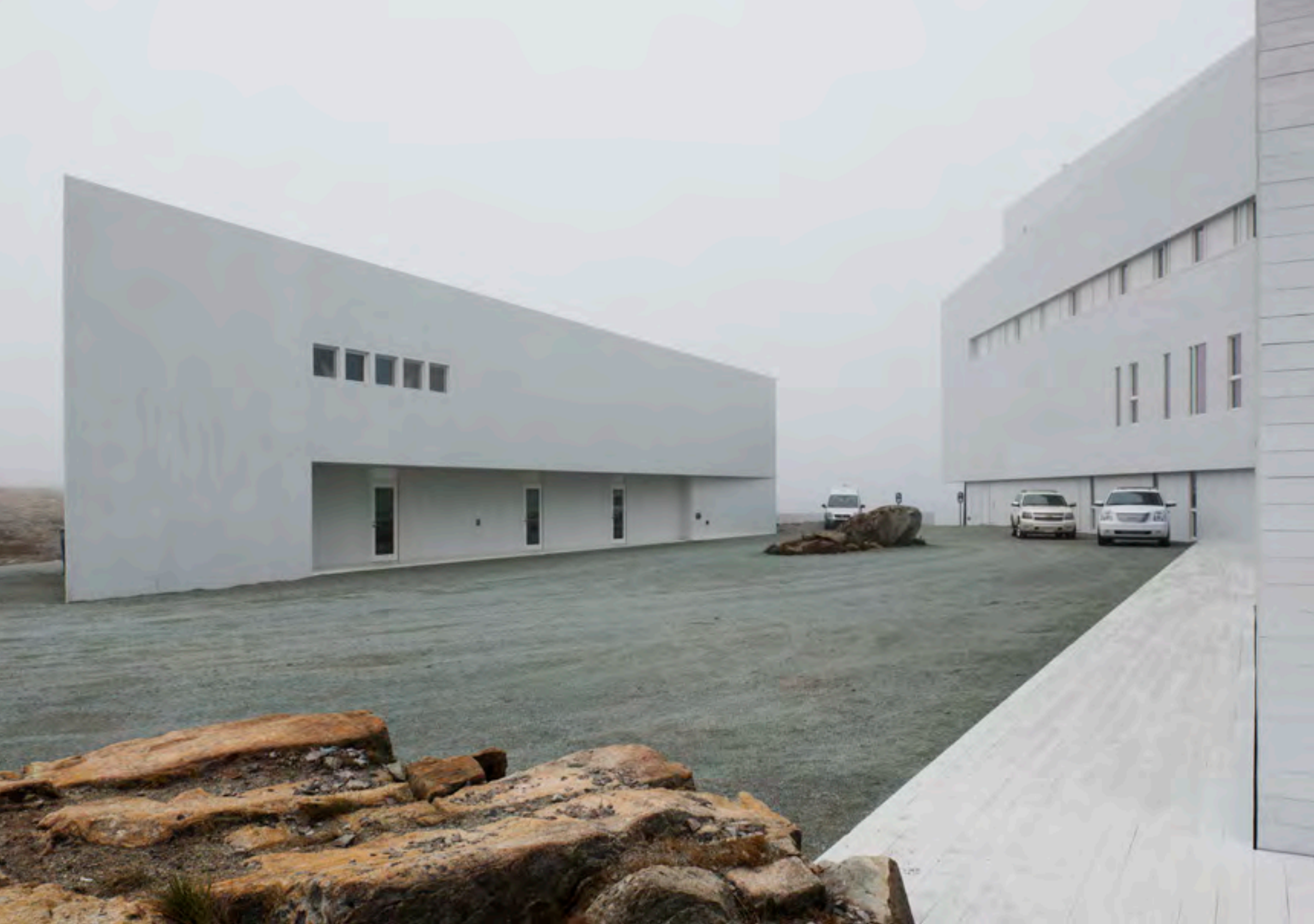
The outbuilding and entrance courtyard / FII_Architecture_6493_photo_Alex_Fradkin
