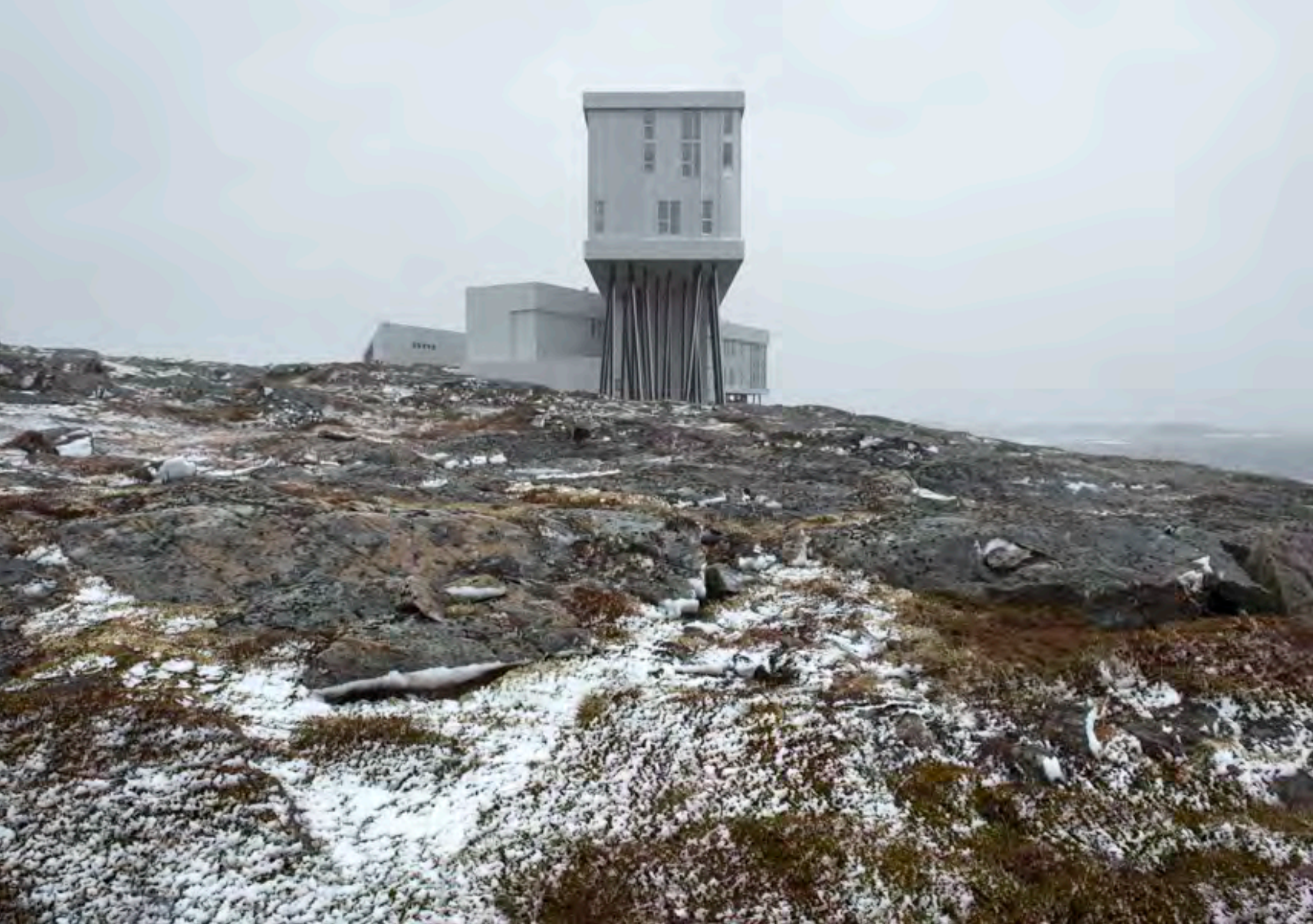
The east facade of the inn / FII_Architecture_3947_photo_Alex_Fradkin
