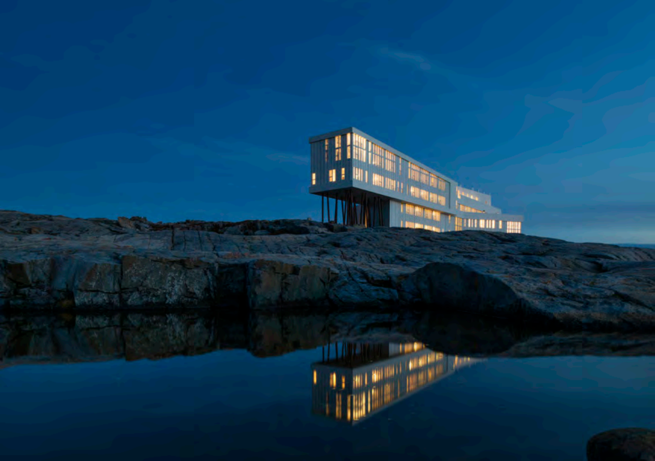
The north and east facades taken from the shore / FII_Architecture_5074a_photo_Alex_Fradkin
