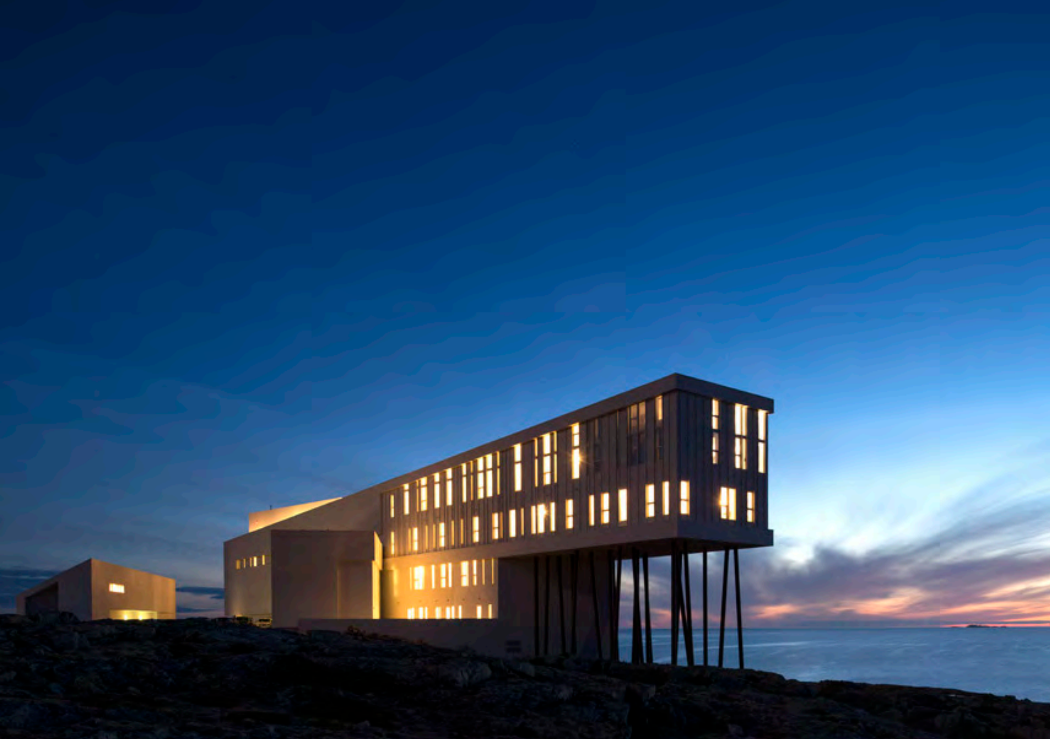
The south and east facade. The outbuilding is at the far left / FII_Architecture_5092_photo_Alex_Fradkin
