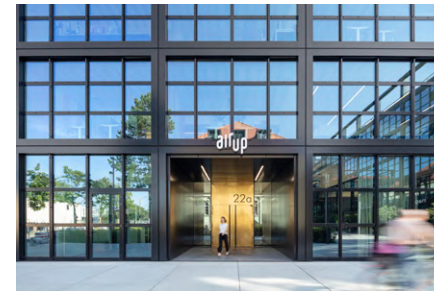
HENN_iCampusRhenania_10 Main entrance (House B) © HGEsch
