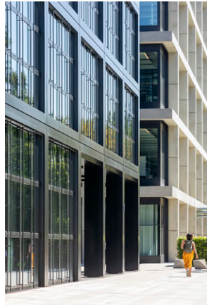
HENN_iCampusRhenania_08 Façade of buildings iCampus Rhenania and House of Communication © HGEsch
