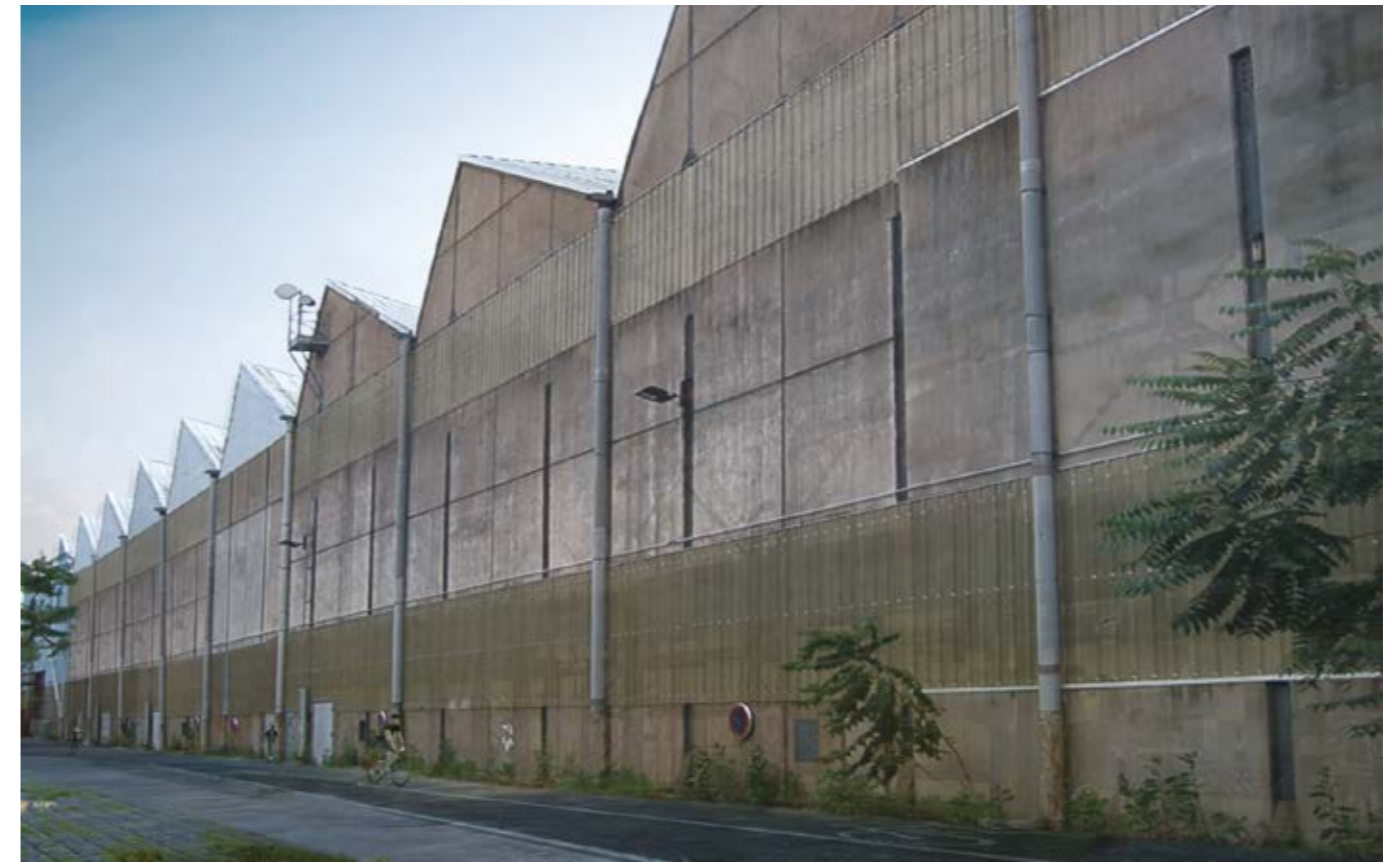
WAREHOUSE N°4 : PICTURE OF THE EXISTING FAÇADE
