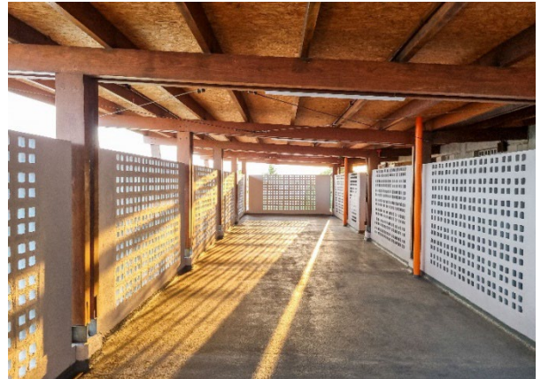
One of the roof terraces
