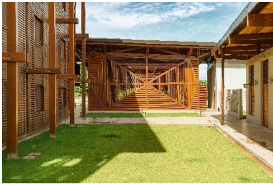
The back wall of the church
