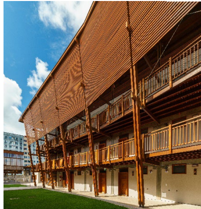
The distribution galleries and brise-soleil
