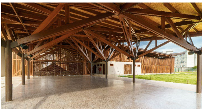
The church square. In the background the church and the refectory
