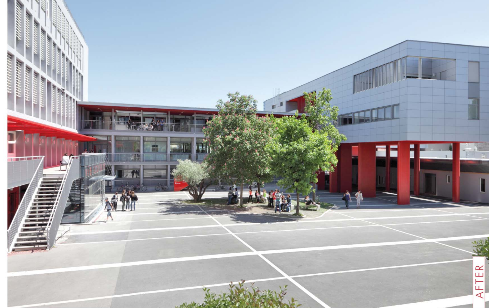
09. Overview of school yard
