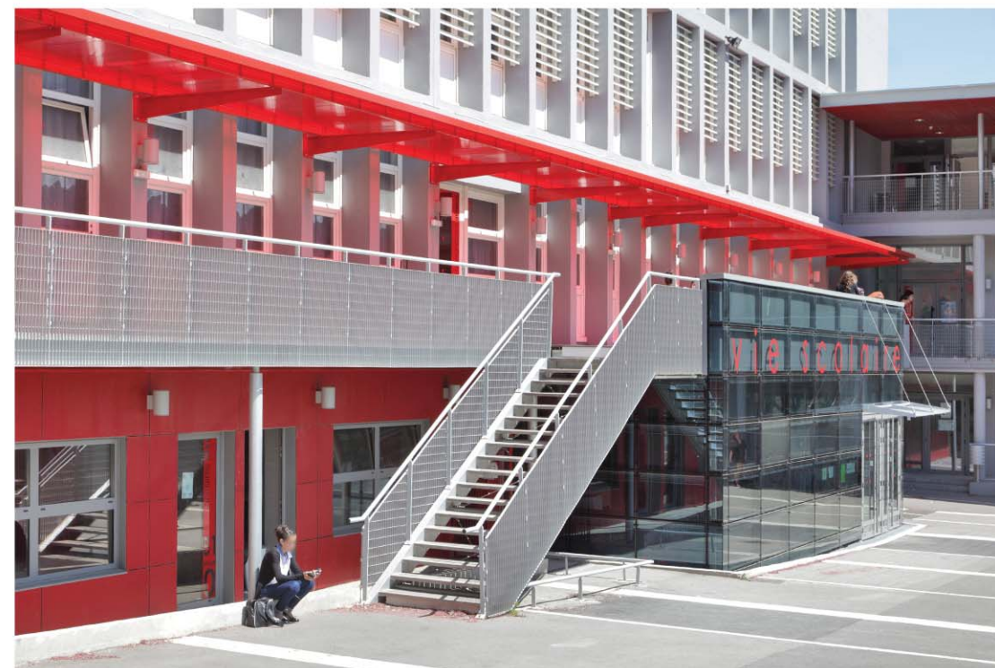
11. A small, entirely glazed central building for school supervisors extends outward from the ground floor courtyard
