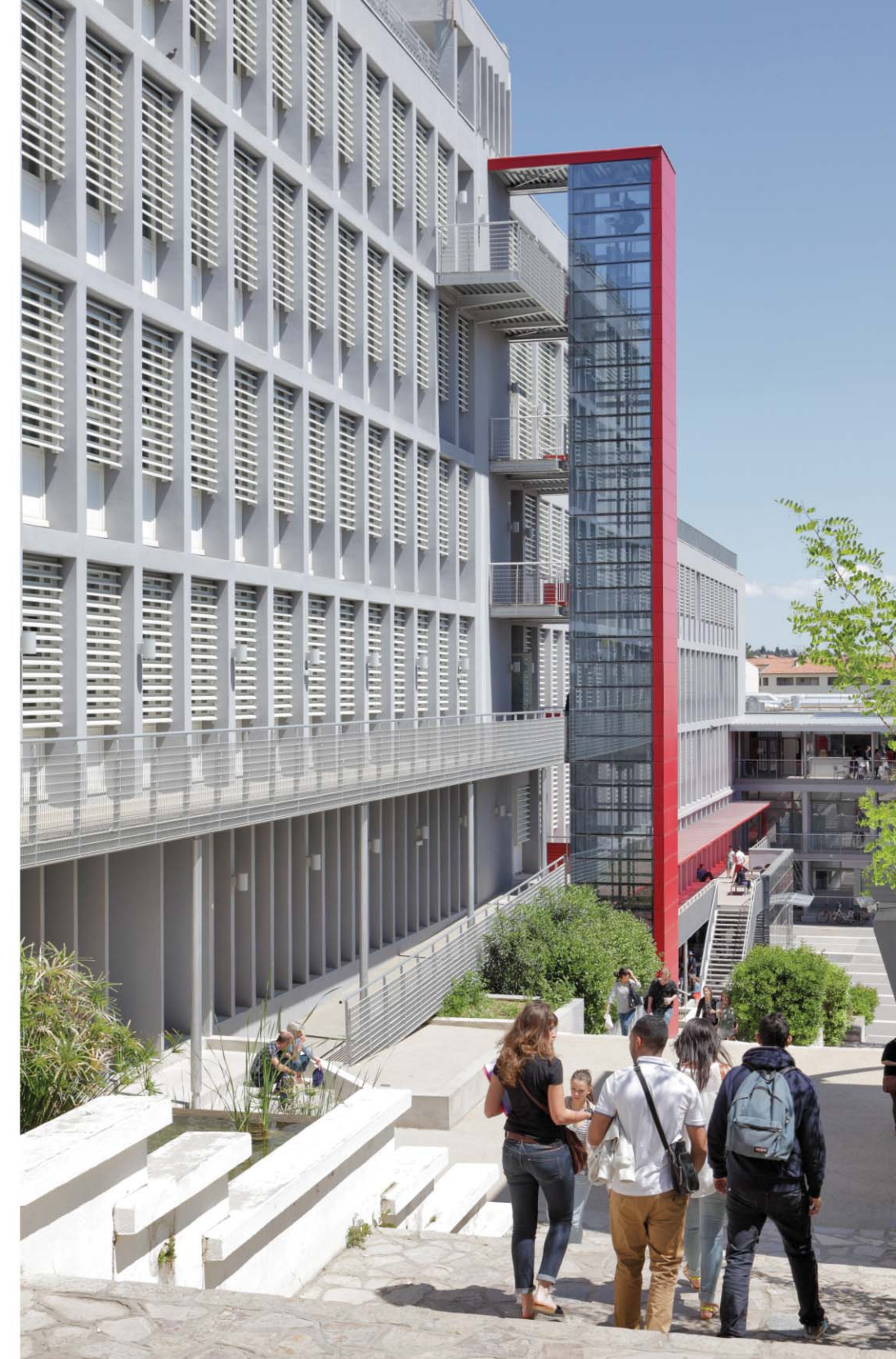
13. The site, view from above
