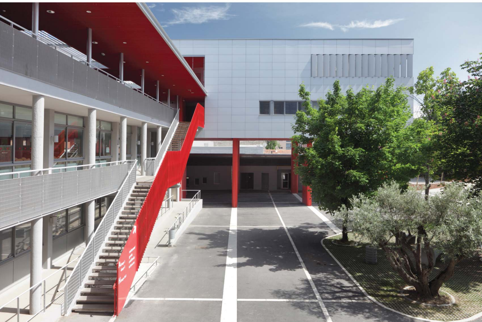
08. Intersection of new STL building and Building A
