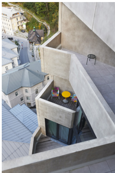
BWM_Bad Gastein_Badeschloss_Facade Detail 03 ©BWM_Designers & Architects_Lukas Schaller
