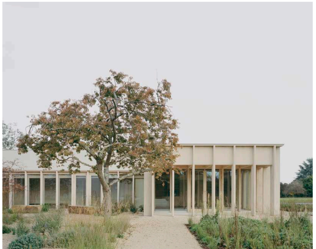
RIGHT Public entrance foyer, constructed in Siberian Larch glulam.
