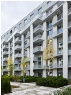
Freilager Albisrieden, Südhof, Zürich Zürcher Freilager AG 270 apartments Invited competition, 1 st Prize 2010 – 2016
