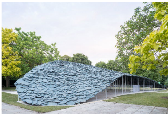
Serpentine Pavilion 2019 Designed by Junya Ishigami
