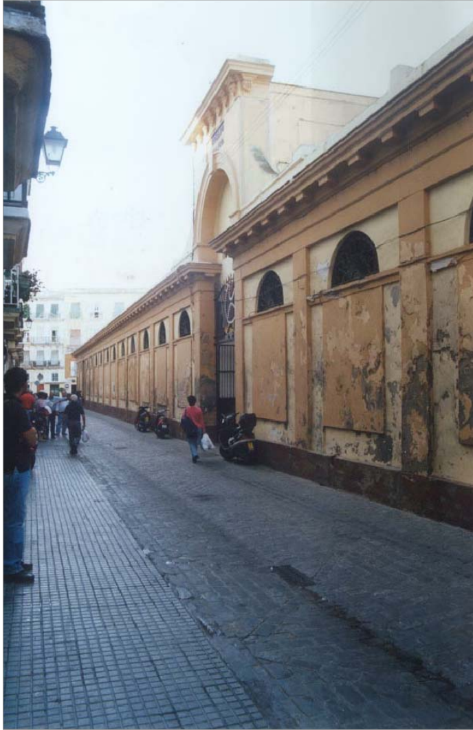
OLD BUILDING EAST FACADE BEFORE INTERVENTION
