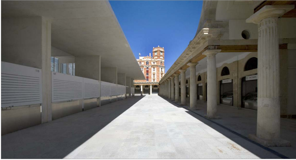
INTERNAL STREET IN BETWEEN THE OLD AND NEW BUILDINGS
