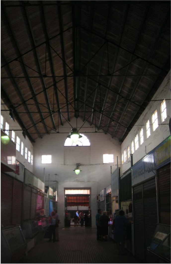
OLD BUILDING CENTRAL GALLERY BEFORE INTERVENTION
