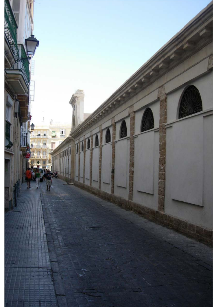
OLD BUILDING EAST FACADE AFTER INTERVENTION
