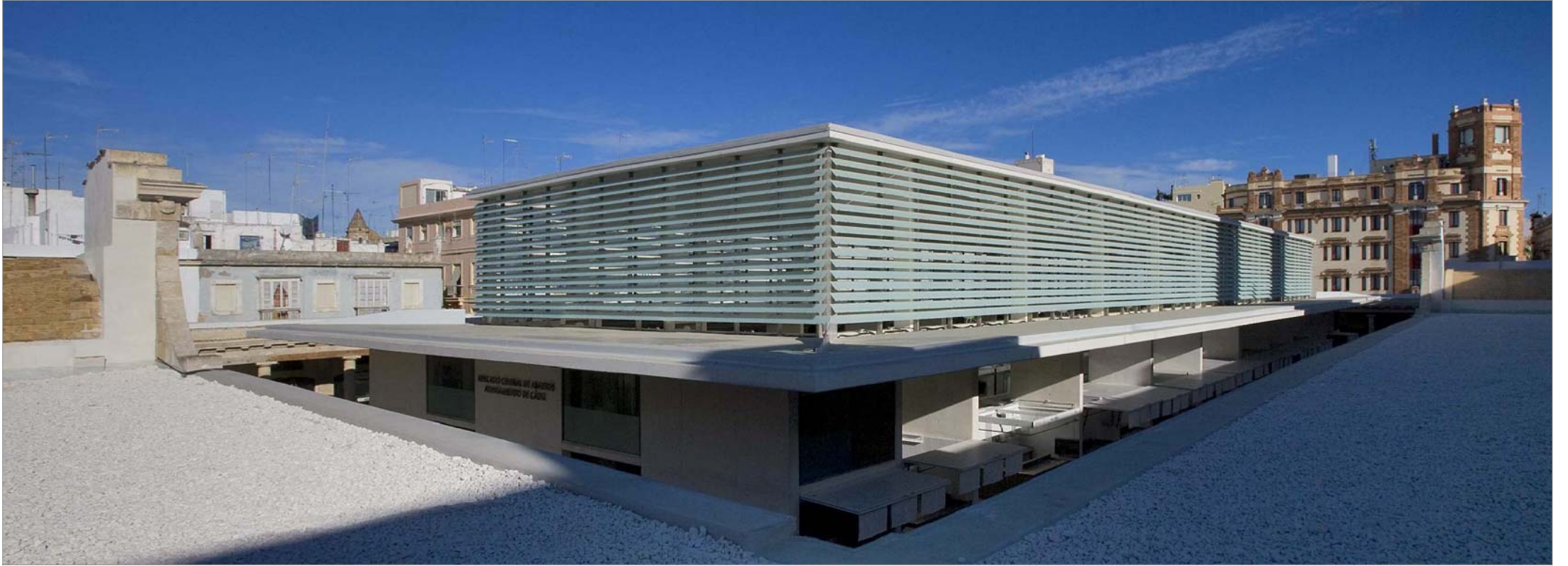
CENTRAL VOLUME FROM THE EXISTING BUILDING ROOFTOP
