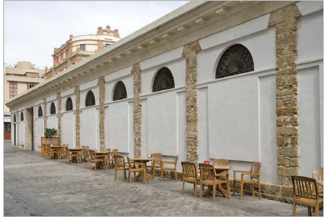
OLD BUILDING WEST FACADE AFTER INTERVENTION
