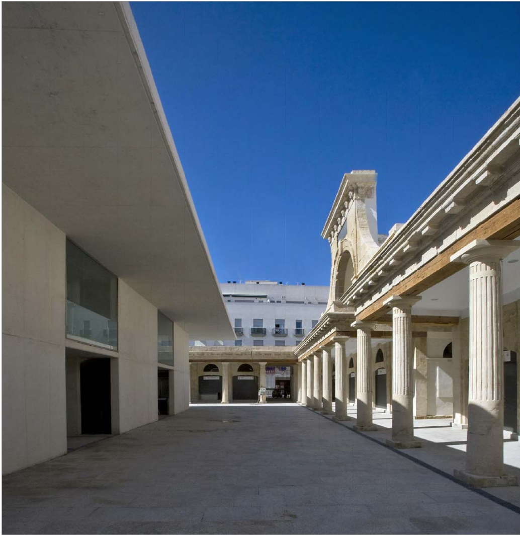
INTERNAL STREET IN BETWEEN THE OLD AND NEW BUILDINGS
