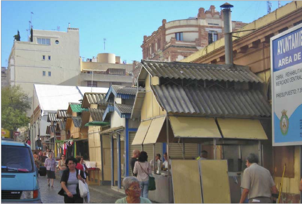
OLD BUILDING WEST FACADE COVERED BY LATER BUILT STANDS, BEFORE INTERVENTION
