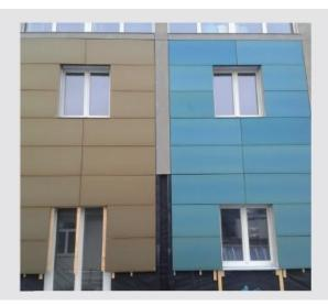
With Kromatix<sup>™</sup> technology, the solar panels are no longer architectural intruders. They can be harmoniously integrated into the building envelope. Roofs, facades and balconies are now fully available to collect the sun radiation and maximize the solar energy production.
