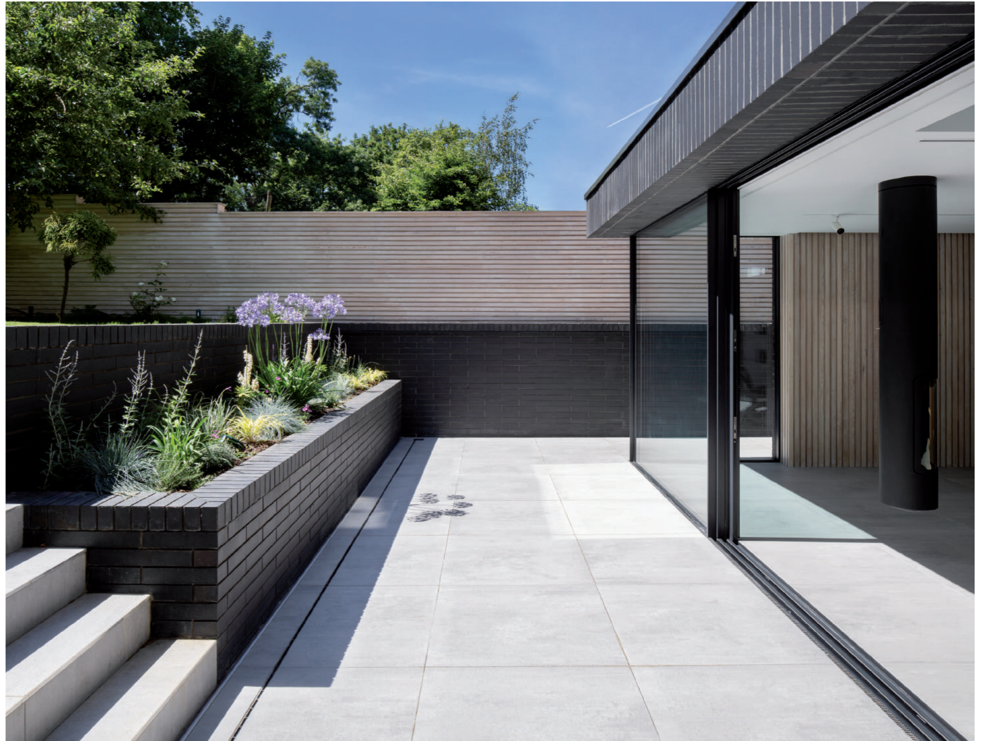
The horizontal stretcher bond linear brick work and larch fence cladding expresses the panoramic horizontal nature of the overall design concept.
