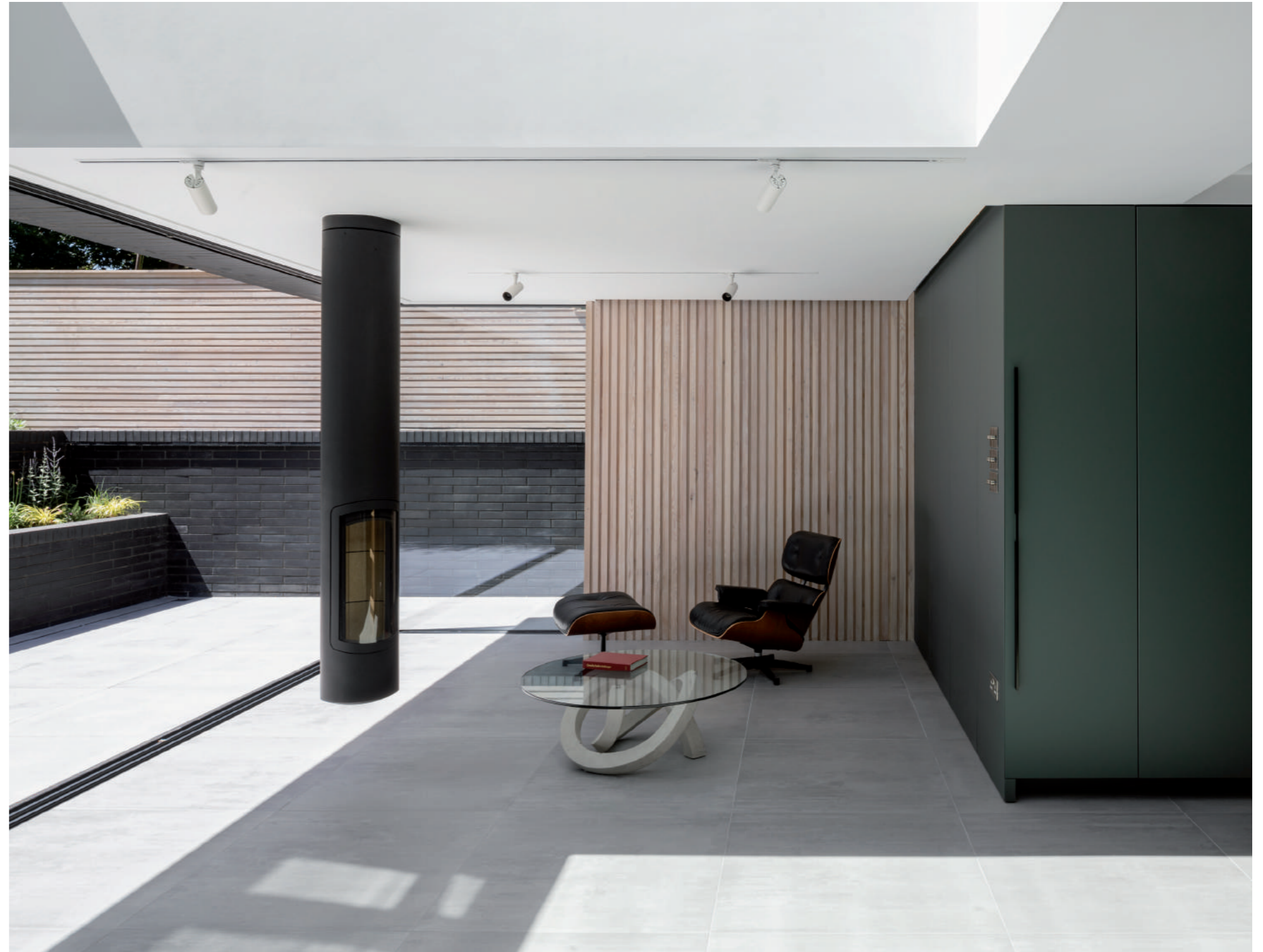
Larch timber batten cladding, finished in white lye oil, is introduced inside and out to compliment the flow of materiality, and mimics the exchange between the vertical (lintel) and horizontal (wall) orientations seen in the brickwork.
