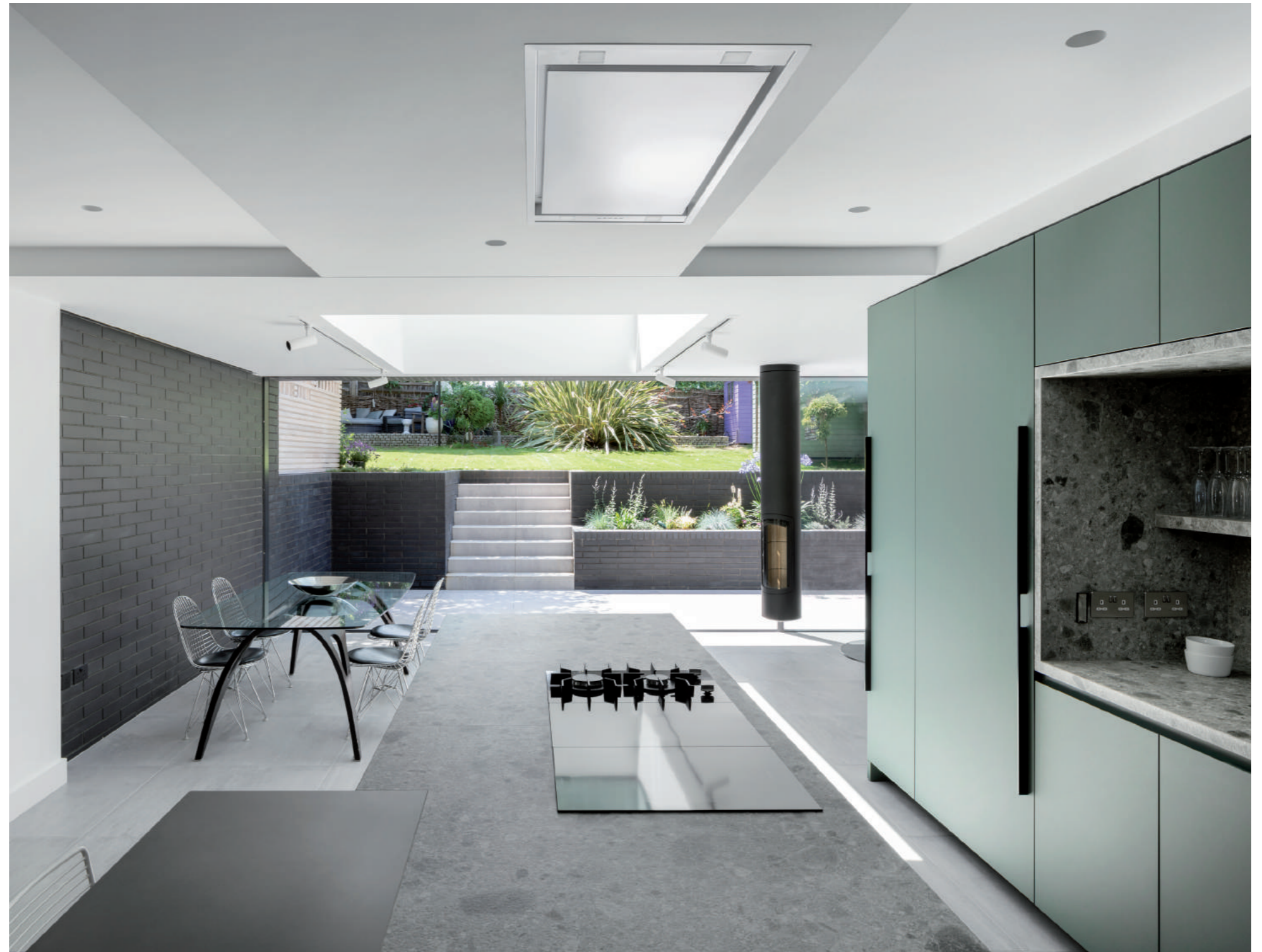
The ceiling plane is carefully designed and co-ordinated with concealed services, lighting and structure resulting in a crisply detailed part-coffered ceiling.
