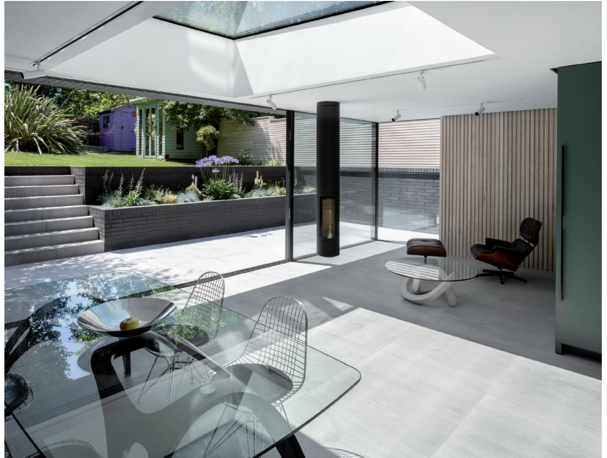
Top light and sky views are enjoyed over the dining area through an oversized 3.5m x 2.4m solar glass single-piece roof light.
