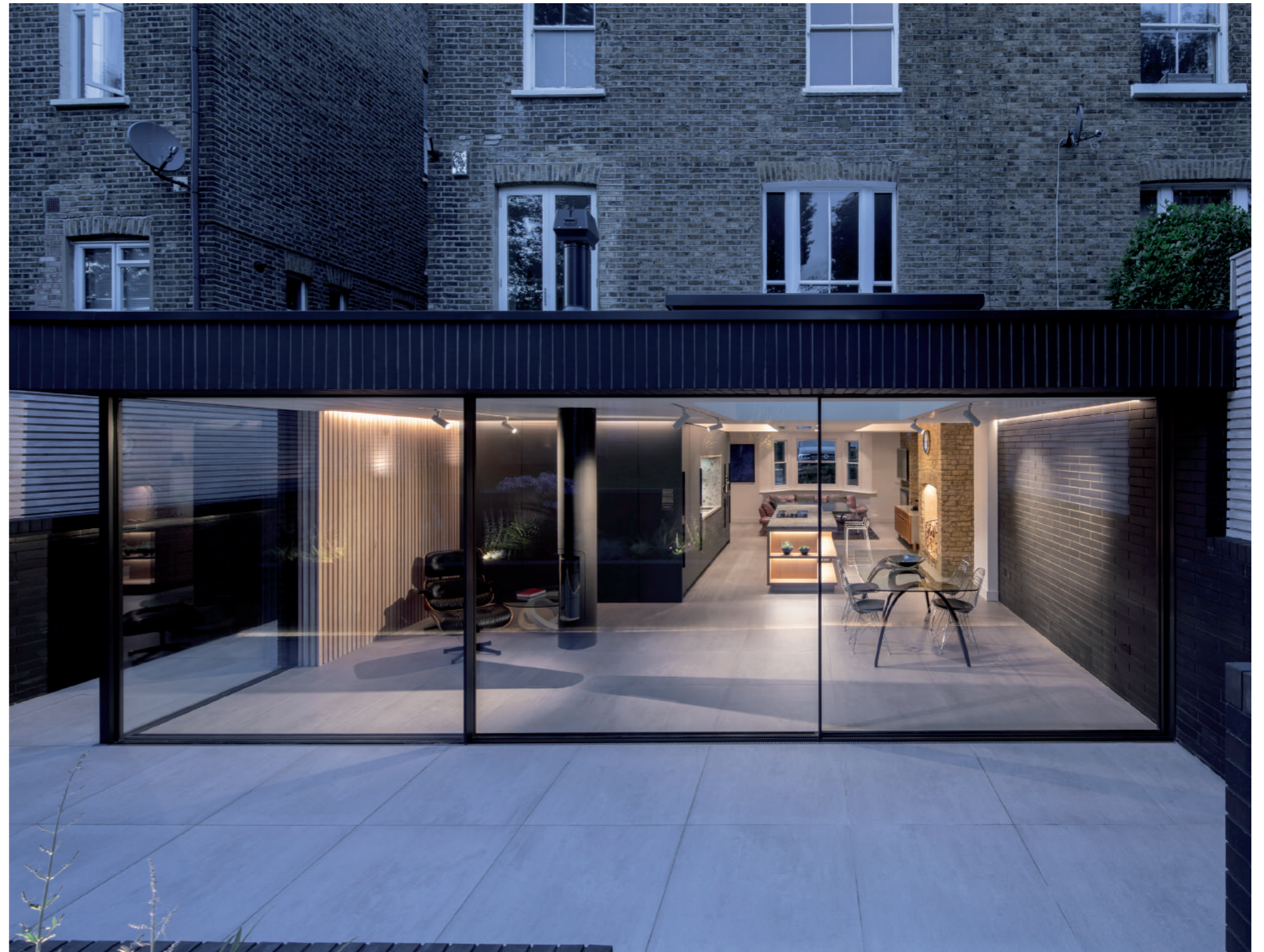
A linear black soldier course brick forms the wrap around lintel to the slab-like roof, designed to appear heavy, yet hovering above the thin framed glazing below.
