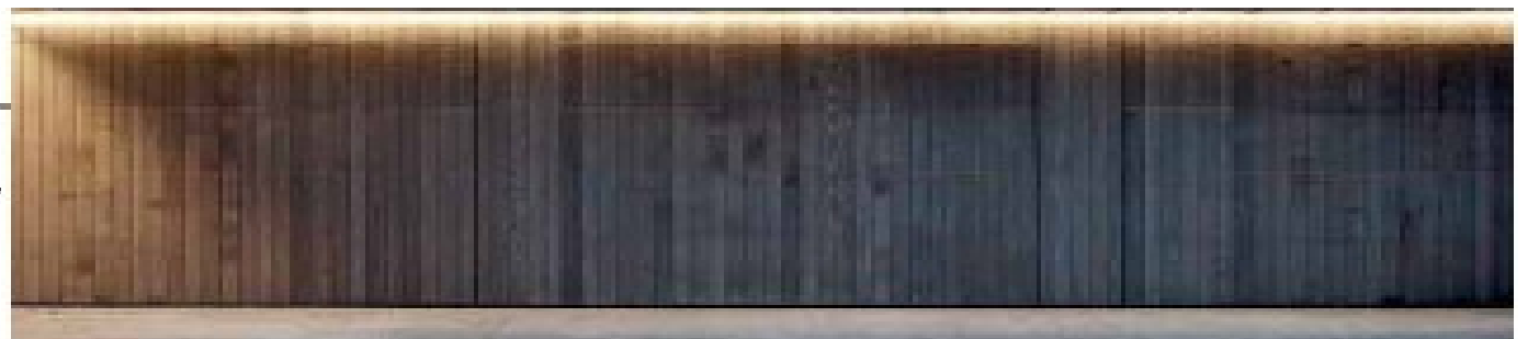
Example of wall washed downlight over timber cladding
