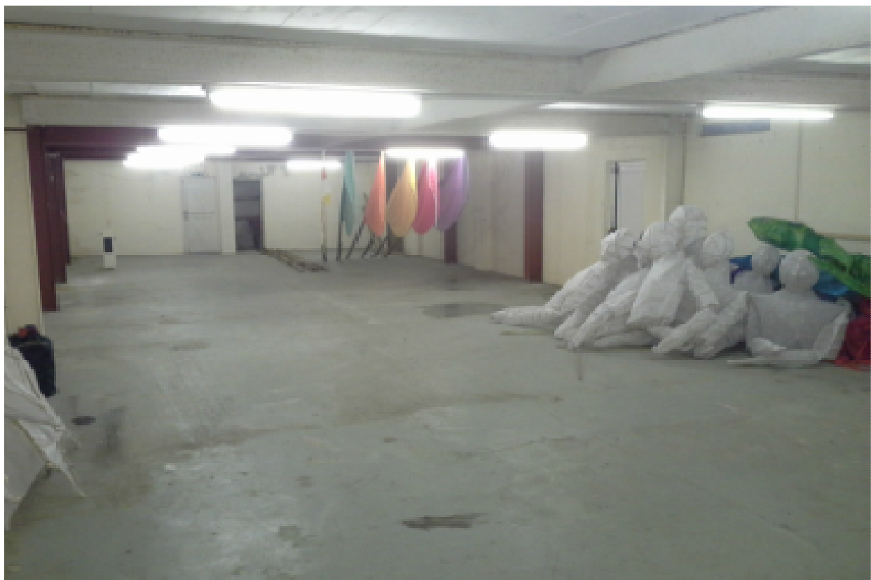
Existing Interior View of Changing Rooms
