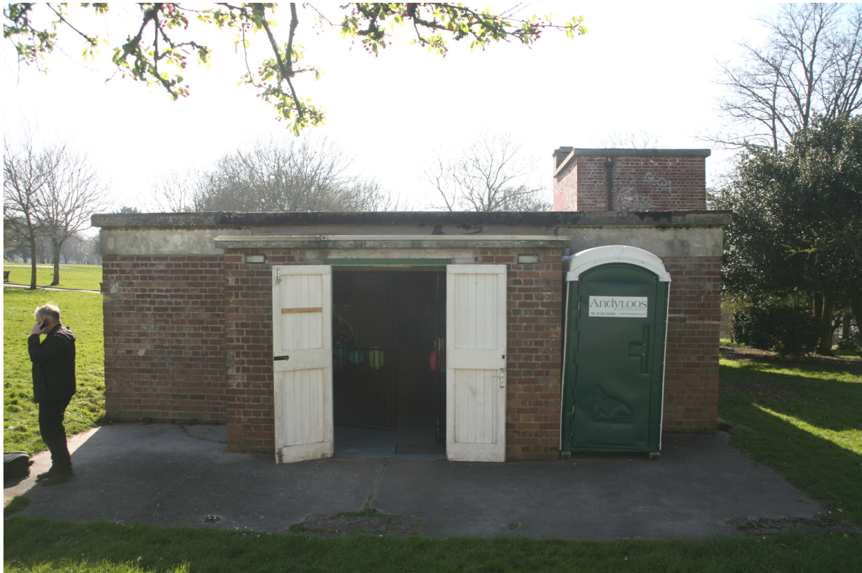
Existing East Entrance Elevation of Changing Rooms
