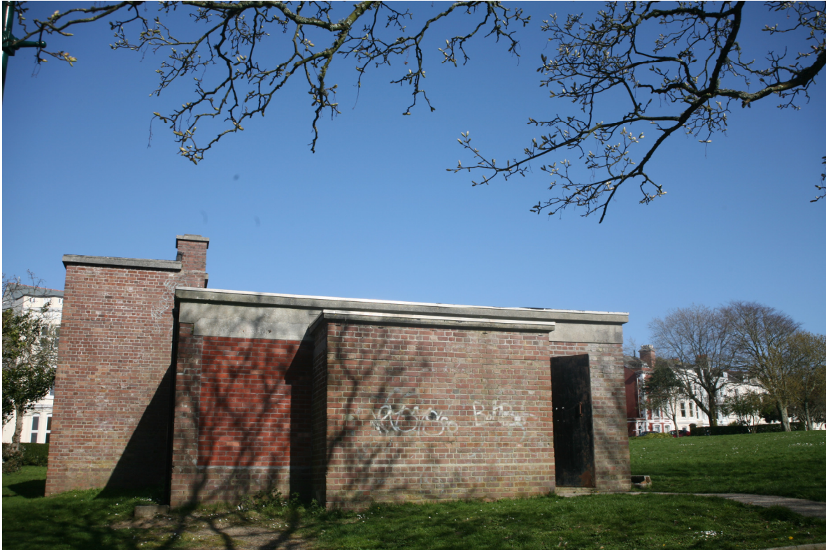
Existing West Elevation of Changing Rooms
