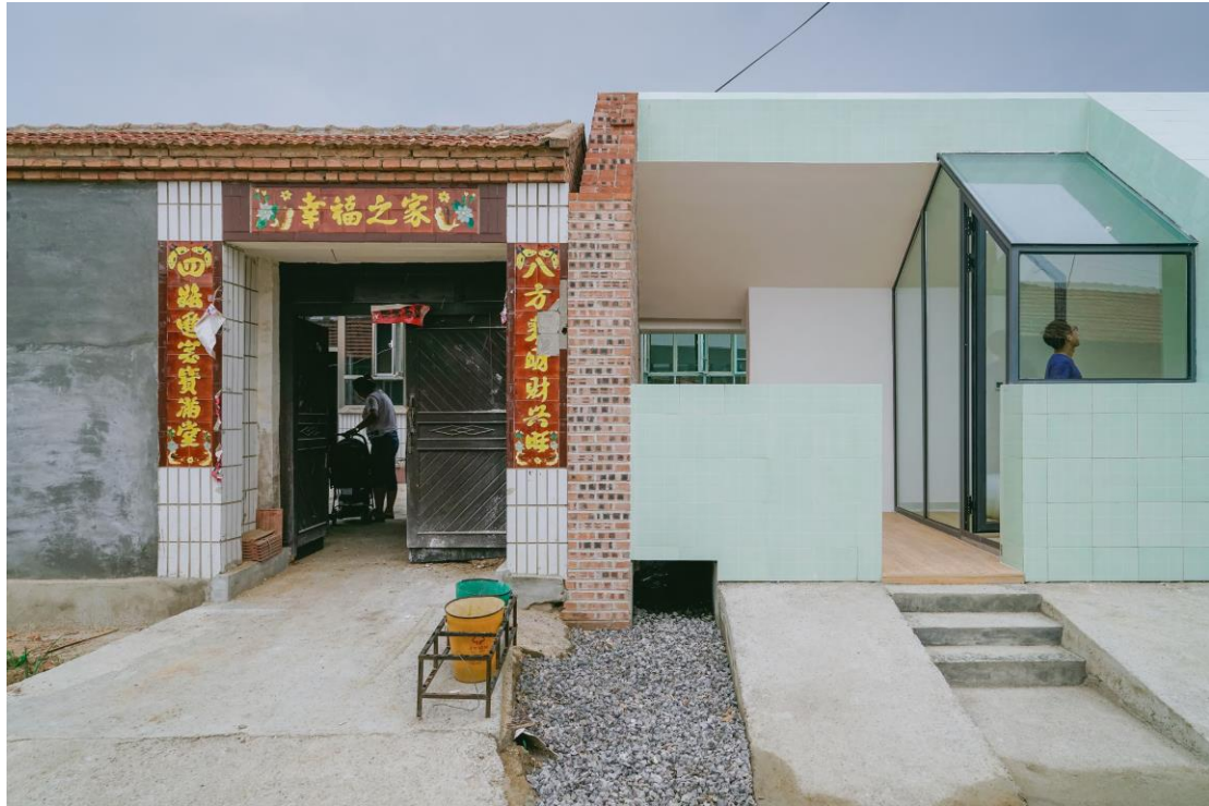
水泥、砖块、铝合金和瓷砖构成了华北乡村的典型建材 Cement, bricks, aluminum alloys and ceramic tiles constitute the typical building materials of the North China countryside
