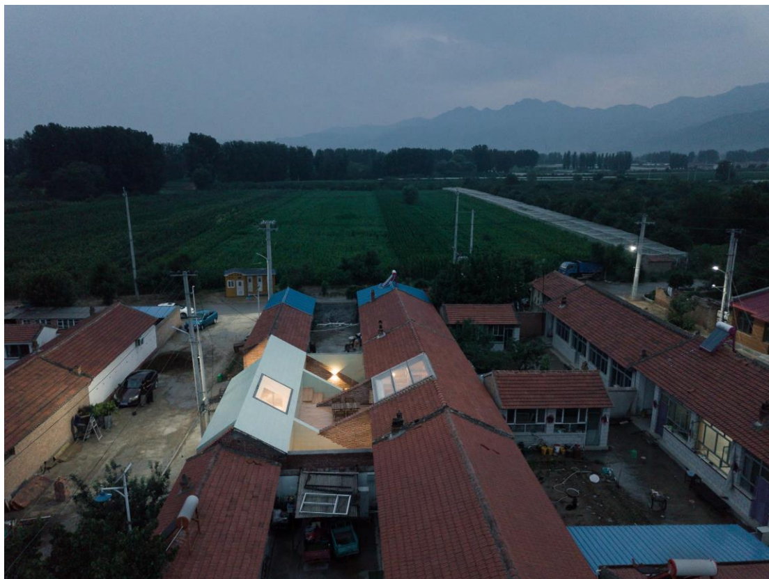
南侧新房与北侧老屋产生对话，两者形成“互”字般的咬合扣接 The new house on the south side and the old house on the north side have a dialogue, and the two form a "mutual" occlusion.
