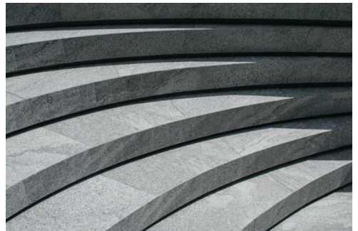
CAR PORCH ENTRY STEPS BLEND INTO LANDSCAPE
