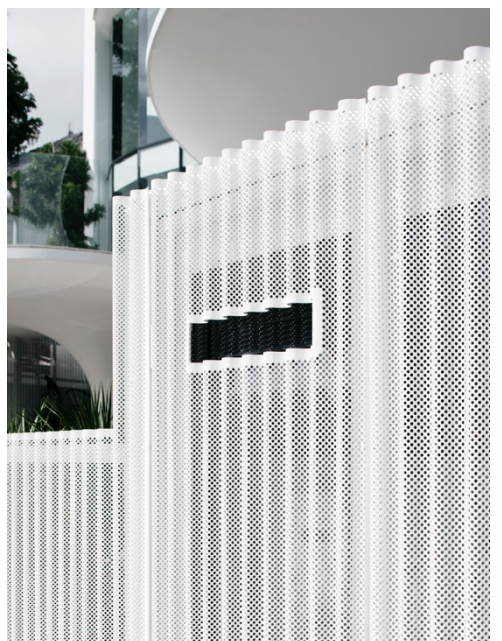
CORRUGATED PERFORATED FRONT GATE AND BOUNDARY WALL
