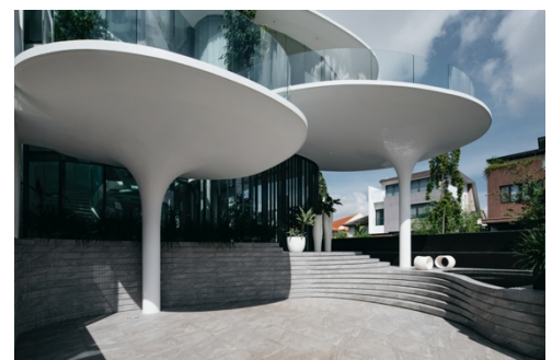
CAR PORCH AND ENTRY PORCH TO HOUSE
