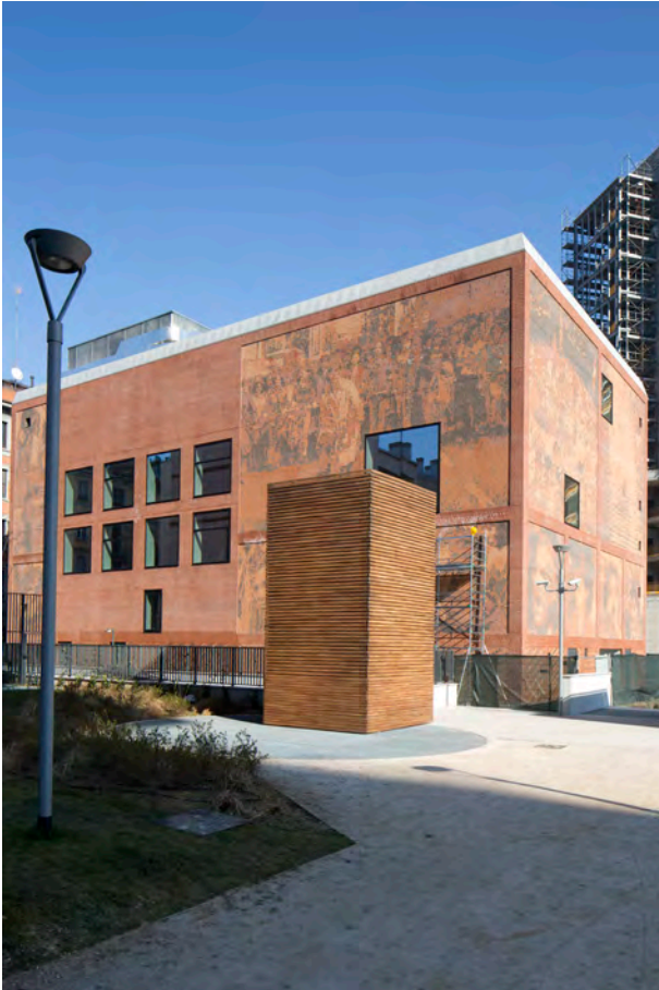
South and west façades (baukuh archive)
