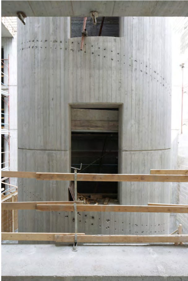
The core of the stairs during construction (© Stefano Graziani)
