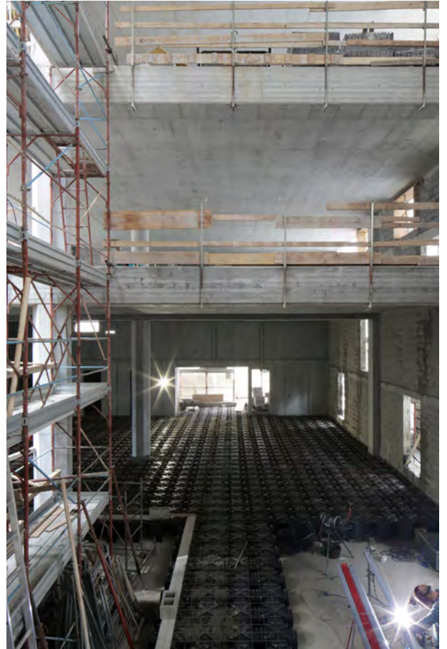
Inside of the building during construction (© Stefano Graziani)
