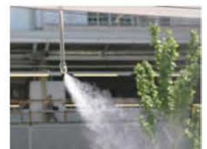
View of mist cooling system
