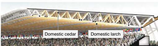
View of using lumber for the truss of the Large Roof
