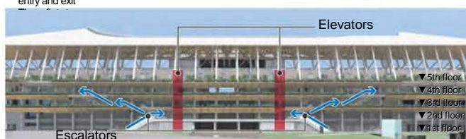
Safe travelling between layers by using elevators and escalators
