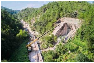
Construction in Quarry #10, photo: Wang Ziling © DnA_Design and Architecture
