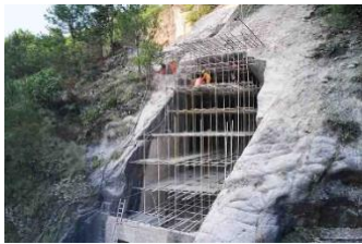
Construction in Quarry #8, photo: Wang Ziling © DnA_Design and Architecture
