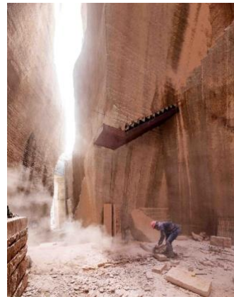
Construction in Quarry #8, photo: Wang Ziling © DnA_Design and Architecture
