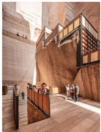
Quarry #8 finished, photo: Wang Ziling © DnA_Design and Architecture
