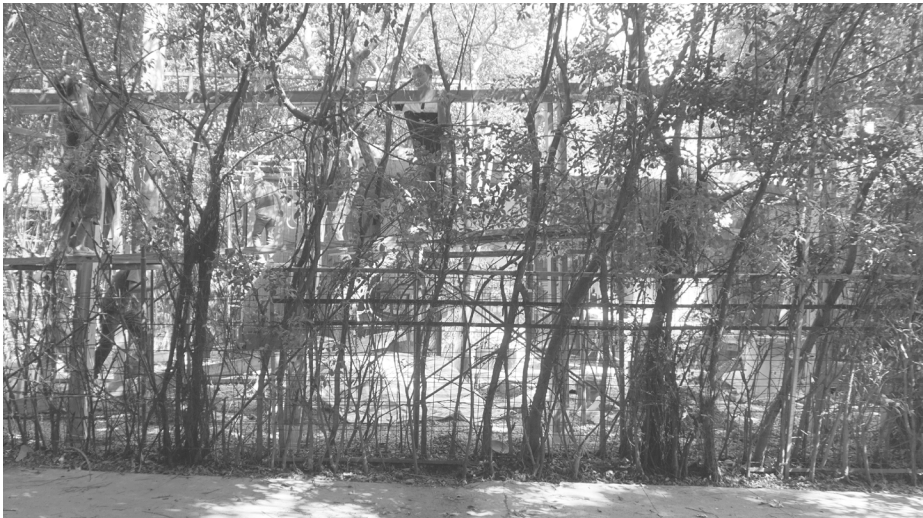
Under-construction, taken in Autumn 2021
