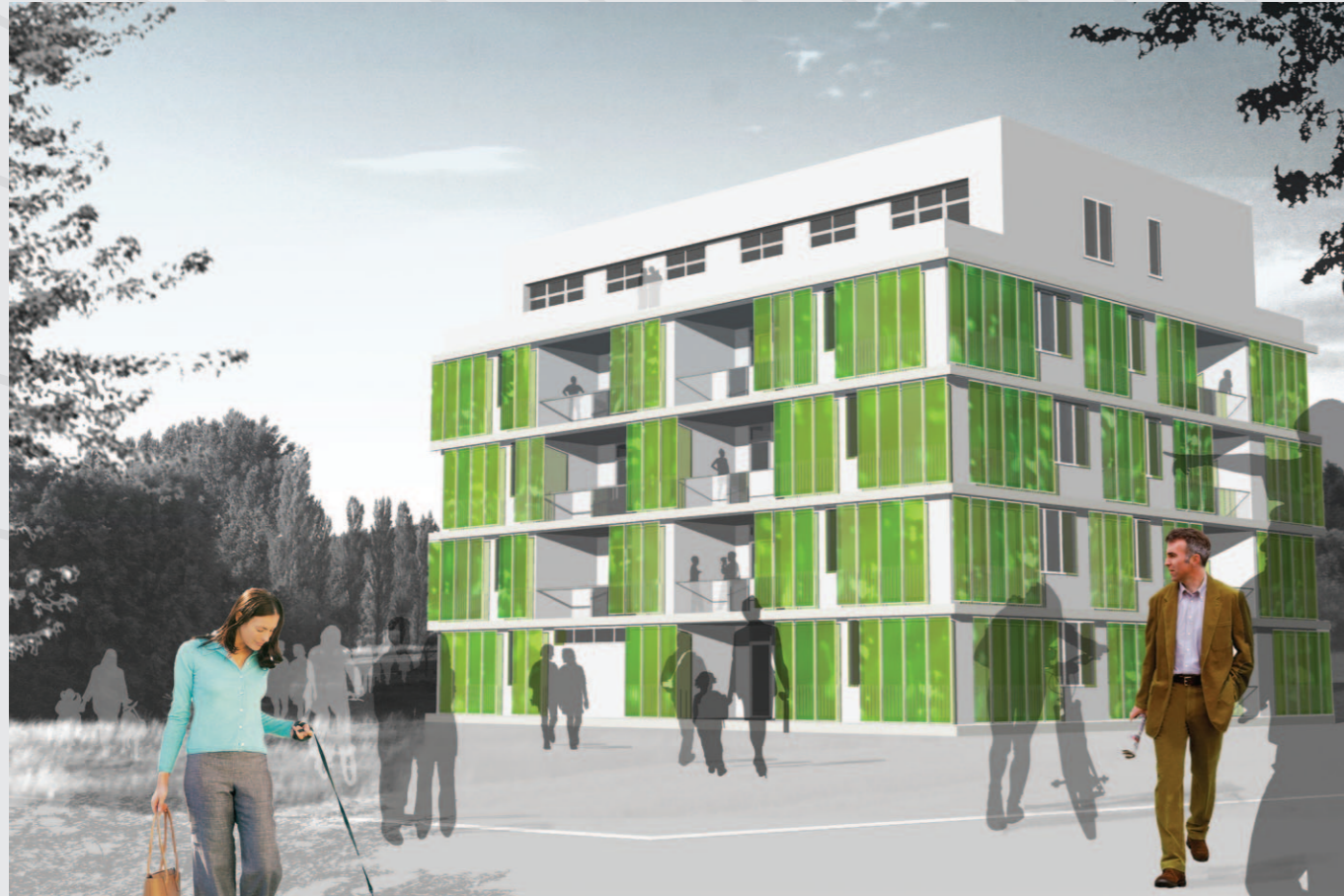
Simulation of the pilot project featuring 200m 2 of PBR for the International Building Exhibition in Hamburg 2013
