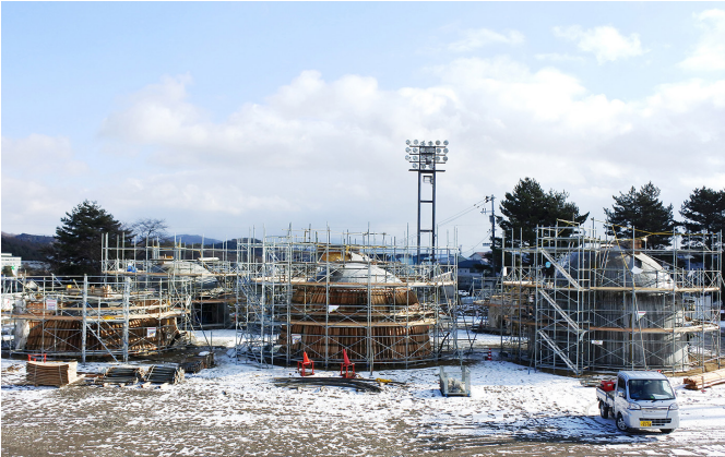
Tamura Indoor Playground Indoor Playground Under Construction
