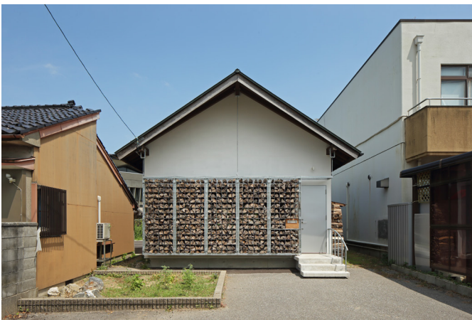
Guest House with Firewood Guest house Completion: 2018
