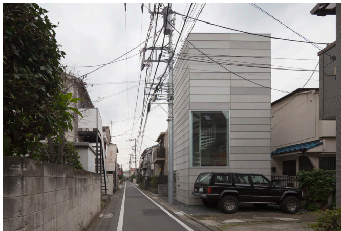
Smallhouse Private Residence Completion: 2010
