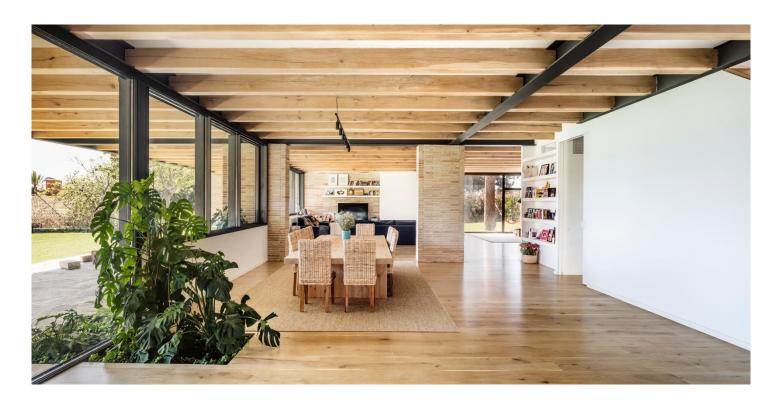
The unity of the brick and its dimensions determine the size of the spaces and the modules of the metal frames that rest on top of the brick walls. This metallic grid modulates the project in an elastic way according to the needs and desired limits. It is a flexible systematization that gives an implicit order to the entire project.
