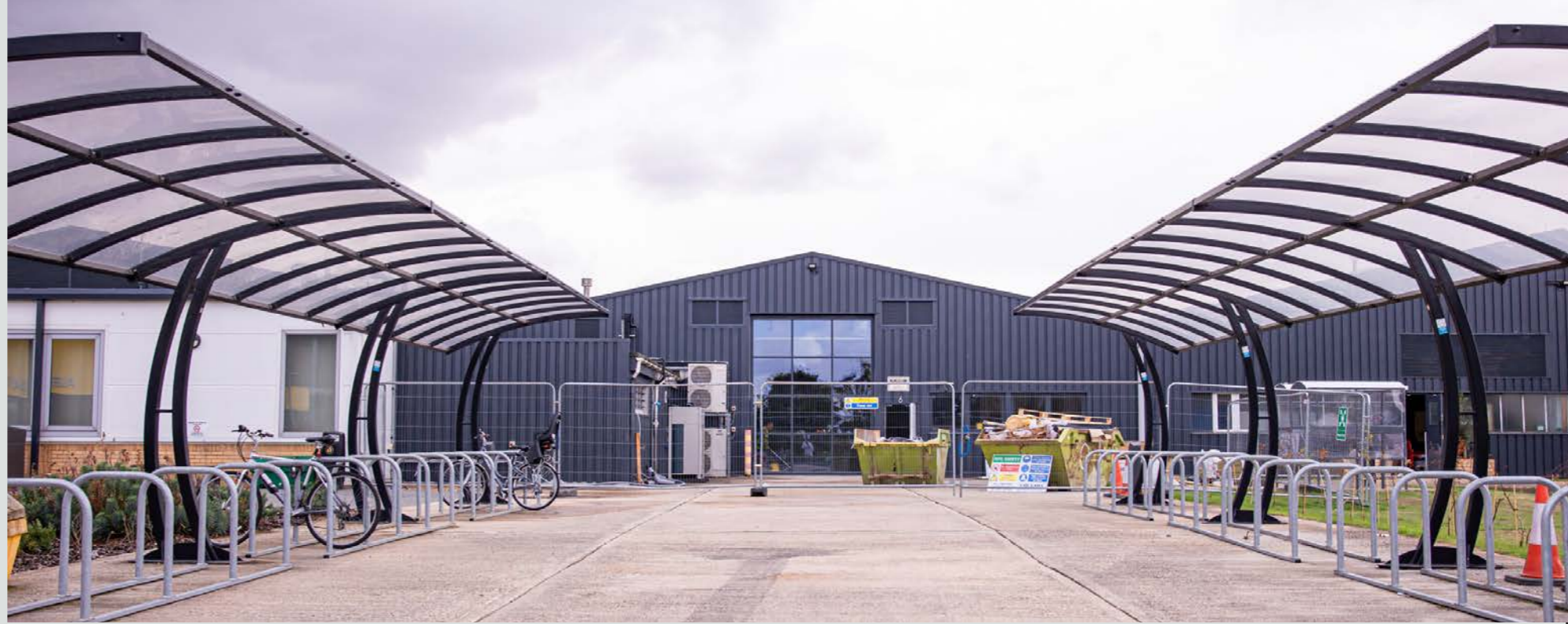
Hangar 02 - External view during construction works
