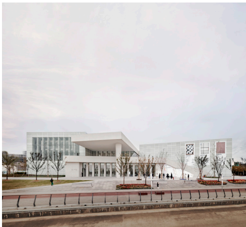
1053_10_SM_191106 East elevation © Simon Menges NO CHARGE
