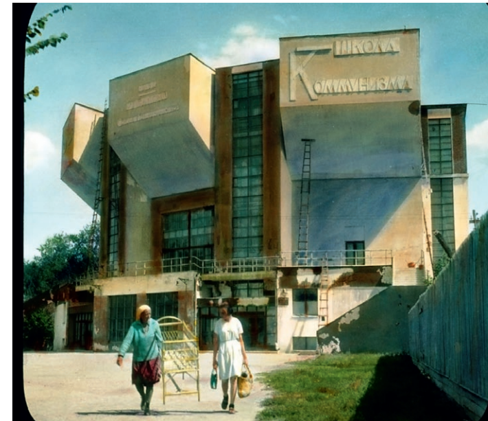
The Rusakov Workers’ Club, designed by Konstantin Melnikov
