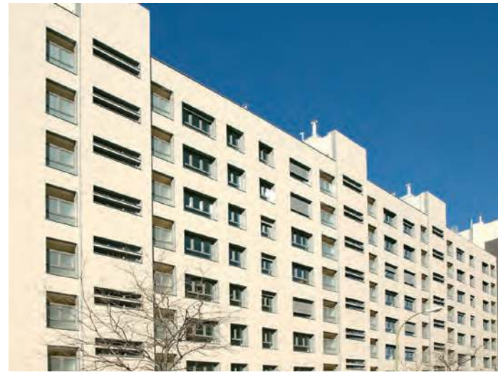
Madrid (SPAIN) Housing block
