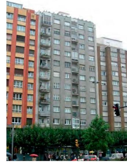
Oviedo (Spain) Housing block
