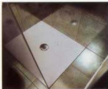
Dettaglio del lavabo con mobile porta biancheria (prod. Ideal Standard). Piatto in vetroresina acrilico (prod. Ideal Standard). Detail of the washbasin with clothes hamper (prod. Ideal Standard). Shower base in acrylic fiberglass (prod. Ideal Standard).
