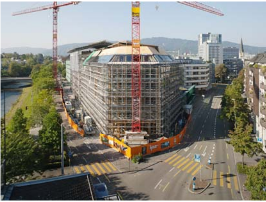
The facade was closed in October 2012.
