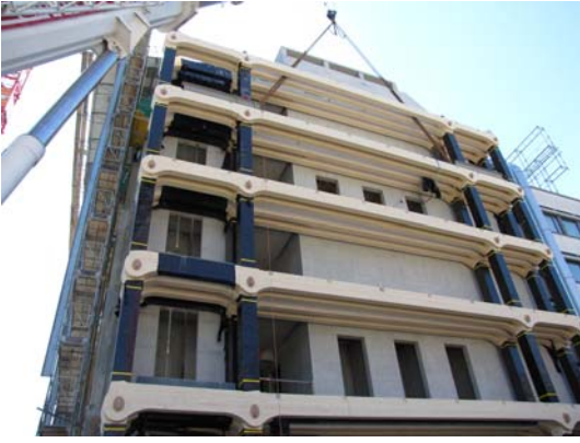
Assembly of the wooden structure began in April 2012.
