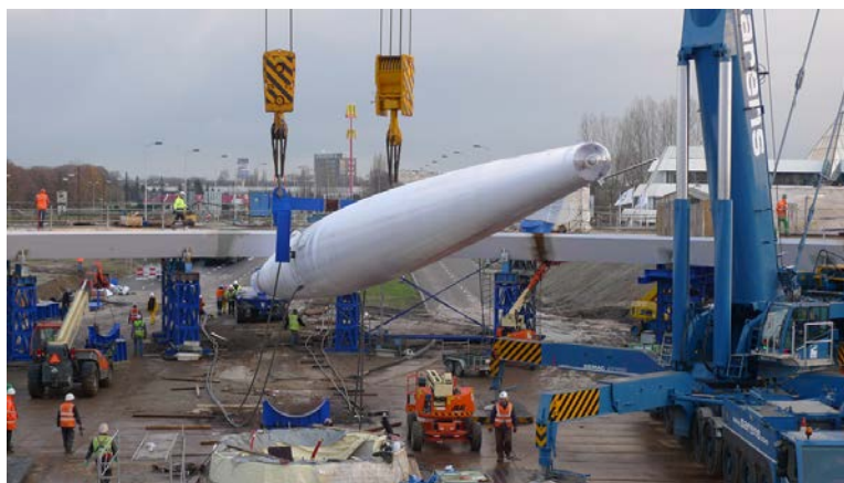
Fig. 9 Construction work on erecting the pylon
