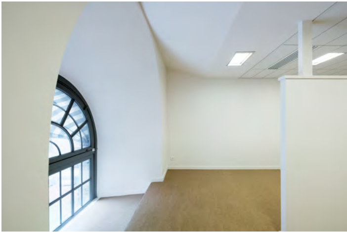
Staging of windows in some offices due to the installation of floors
