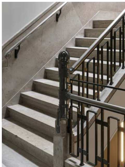
Adapted staircase railing
