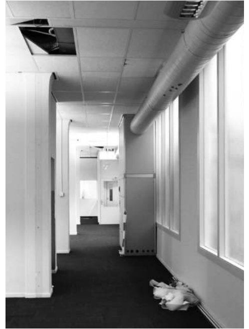
Third floor before the renovation
