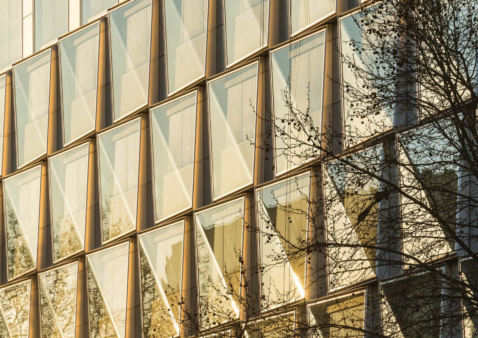
On the garden side, in the heart of the block, wood has replaced aluminum, with blinds in colored canvas being replaced by aluminum strip blinds. From a technical point of view, the solutions proposed have provided better performance than the initial project concept, as the materials used being more resistant to shocks and the wind.
