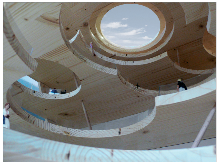
Image 2: Perfectly circular openings in ceilings and floors afford views in and through the large corporate building. They provide many opportunities for employees and visitors to see and meet one another. Users of the building sense its size not only outside, but inside as well. The atriums crisscross the deep and compact building. (Model picture: Christian Kerez)
