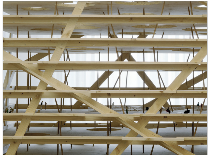
Image 1: The building from the outside, with its interior pillar structure supporting the slabs and the exterior bracing the building as a whole. It enhances the mutually-dependent structures and the relationship which is generated between the building and its industrial landmarks of the surrounding landscape. (Model picture: Walter Mair)
