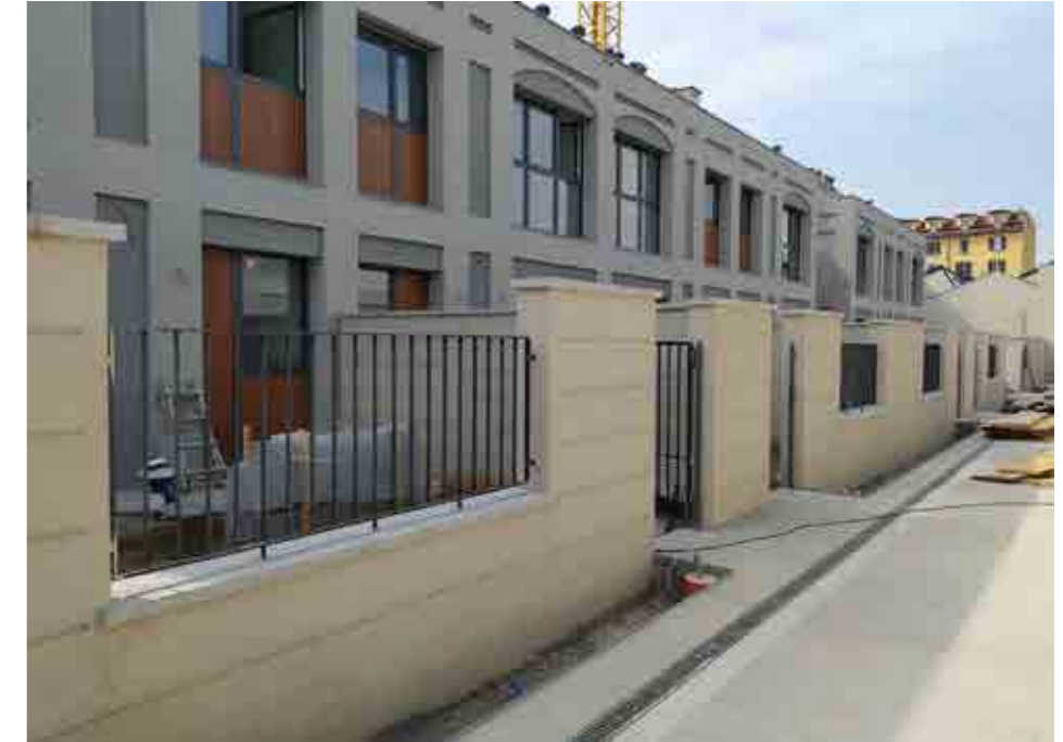
View construction site
