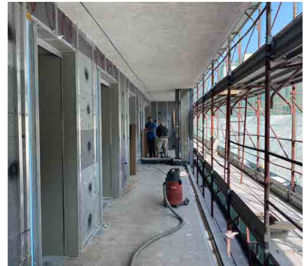
View construction site
