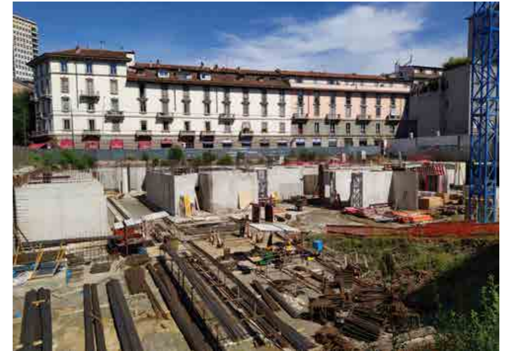
View construction site
