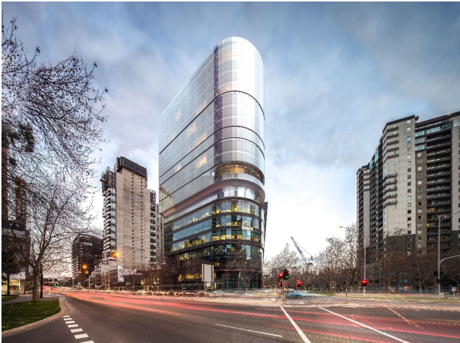
The Adina Southbank Melbourne uses CLT to add 10 levels to an existing commercial building. Image © Bates Smart
