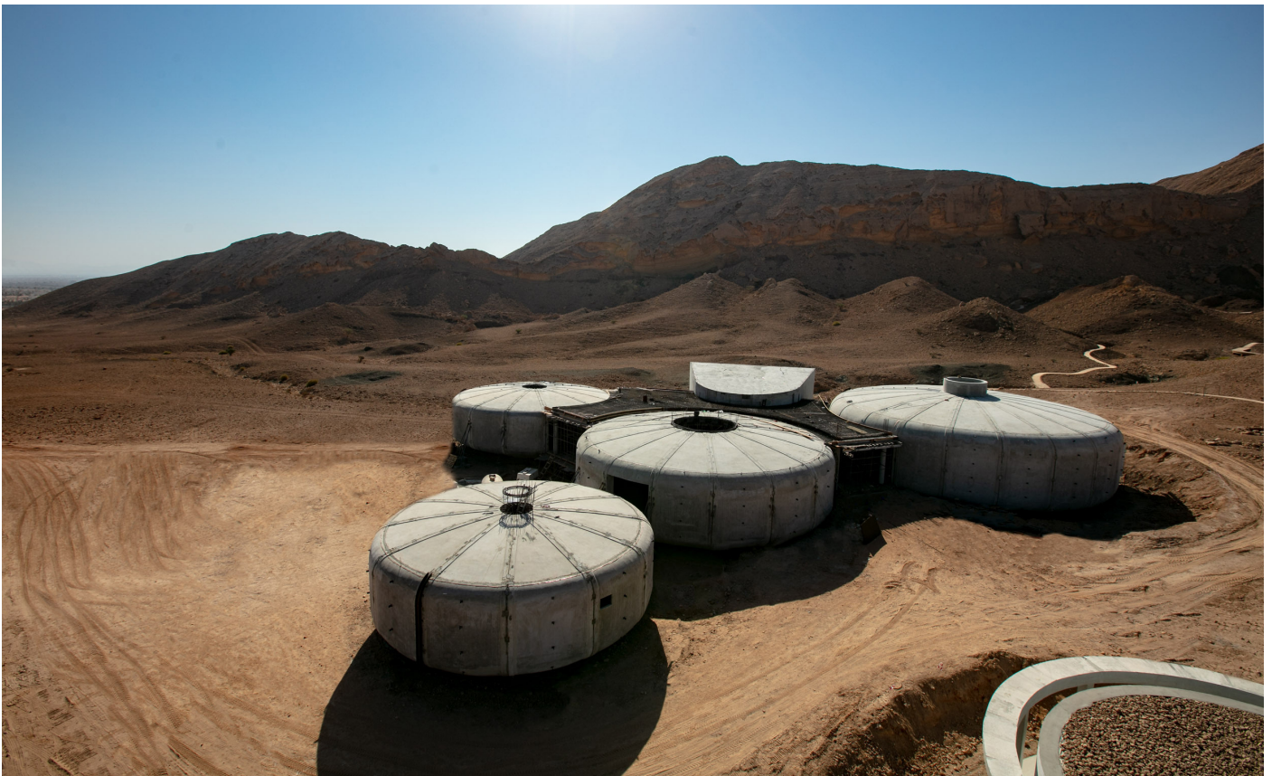
Images of construction process © Hopkins Architects
