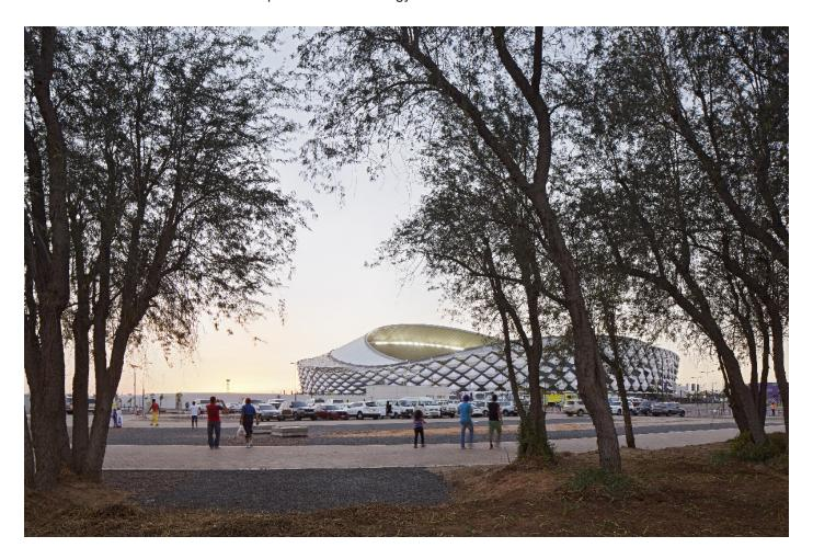
This "Palm Bole" facade also acts as a passive cooling device; shading the building during the heat of the day whilst allowing fresh air to flow. Within the bowl this creates comfortable spectator conditions and aids grass growth for the pitch.
