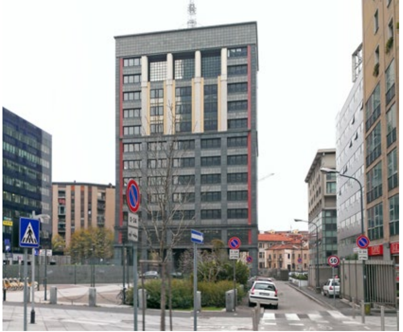
Main elevation - current status
