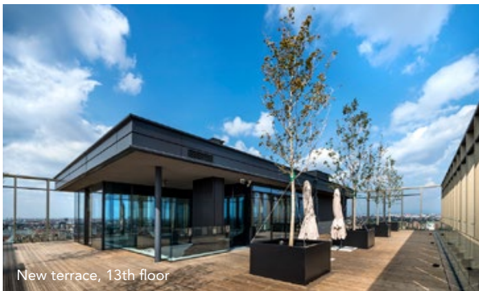
New terrace, 13th floor
