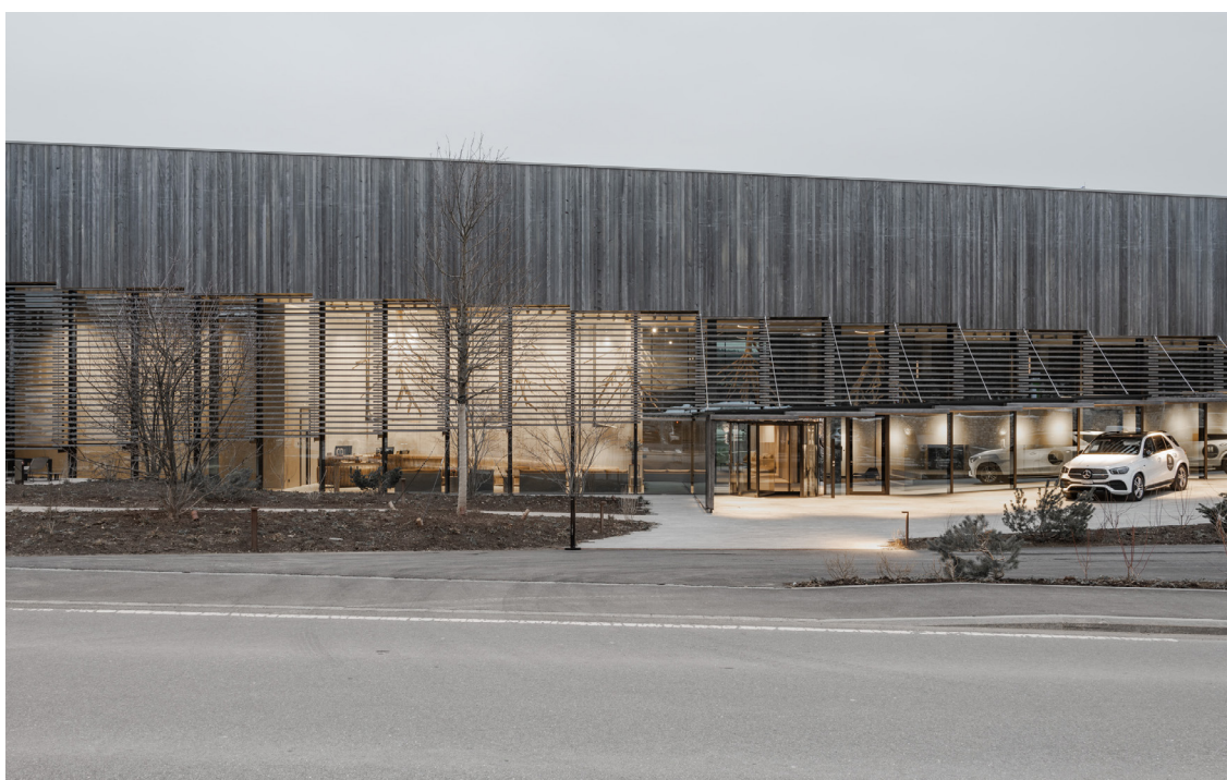
▲ Located on the same site as its predecessors, the new Hôtel des Horlogers perpetuates the long history that began in 1857 with the Hôtel de France – an important stop on the Chemin des Horlogers linking the workshops of the Vallée de Joux to Geneva.
