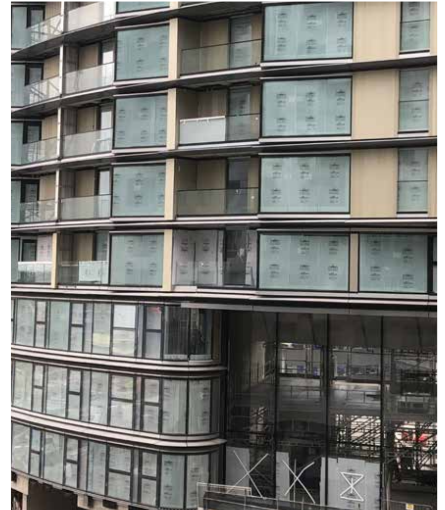
Protec protection sheets used for the building façade
