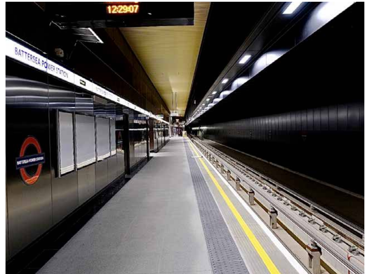
The new Northern line platform at Battersea Power Station
