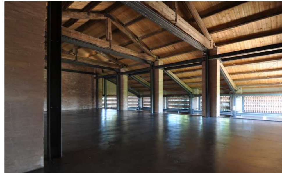
Recovery of the original space, on the upper floor, with the insertion of new metal frames and the recomposition of the external wall tissues ("gelosie") in facing bricks
