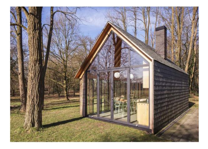
The house has replaced an existing garden house, which foundation is reused and its existing contours were the starting point of the new house. The archetypal cottage is simple: a gable roof of stone slate, a chimney and a wood cladding of Western Red Cedar. The cottage blends into the landscape seamlessly by the natural use of the materials. The architectural drafting, interior design and its realization were in one hand. This has resulted in an unprecedented high level of craftsmanship.
